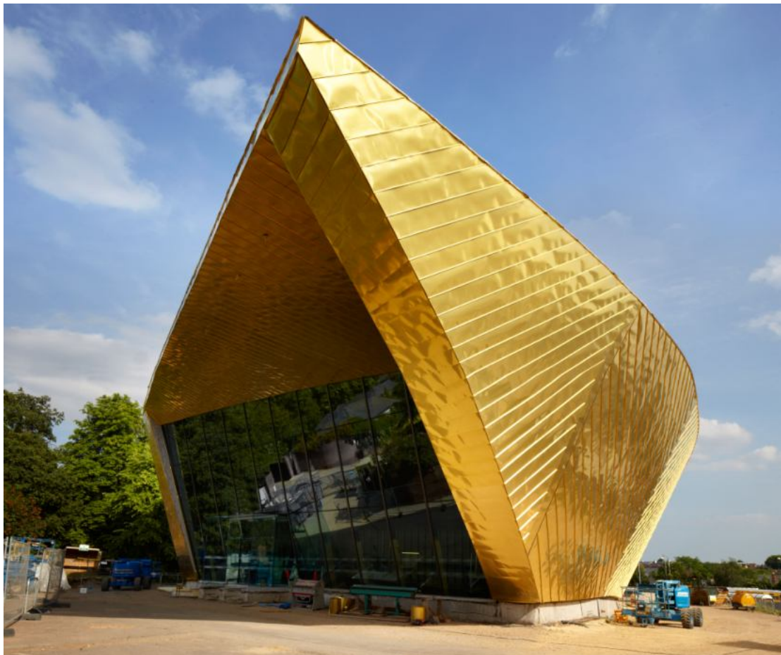
Figure 2 view from below
