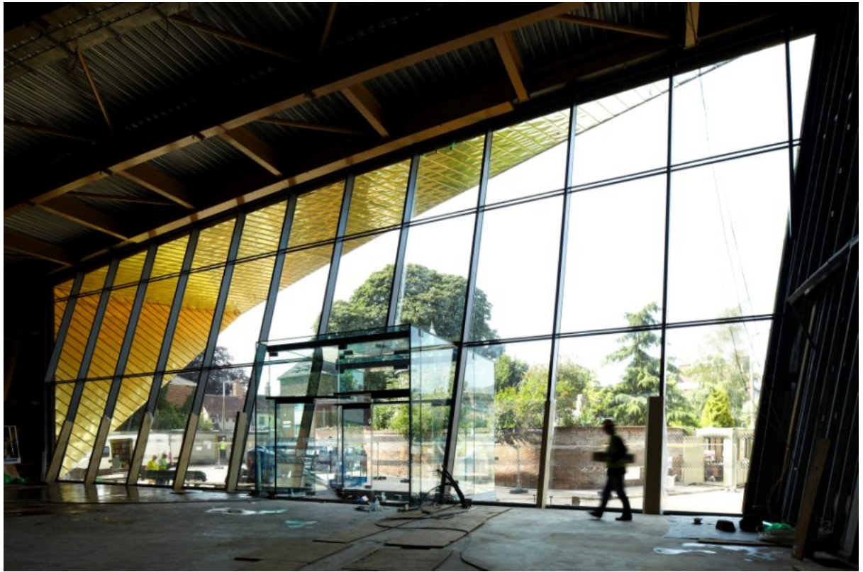
Figure 3 view from inside
