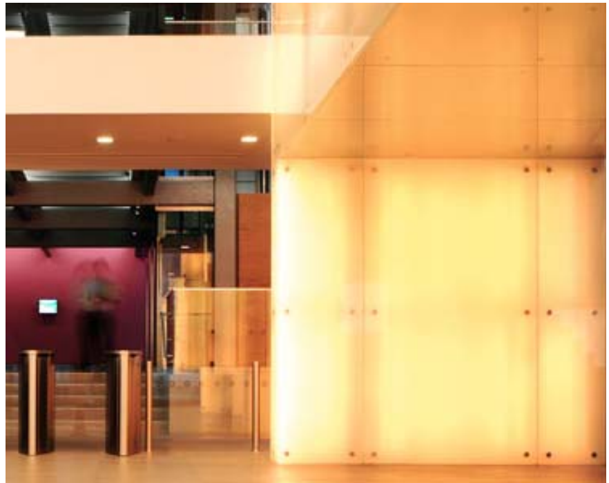
Glass fascia panels (above and below left) add colour and flair to staircase enclosure at offices in City of London
