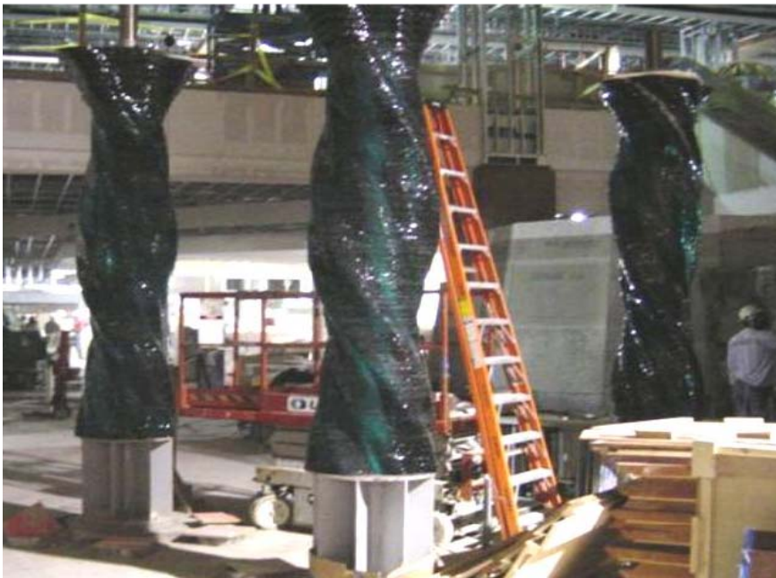
The nine-column glass water feature at Pompano Park in Florida (above). Computer modelling was carried out to ascertain stresses in the solid mass of glass plates (below and left).
