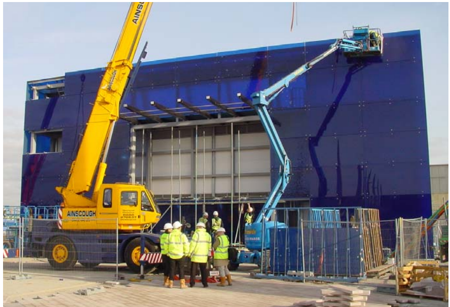
Glass panels provide façade for performance wall at Millennium Sq.
