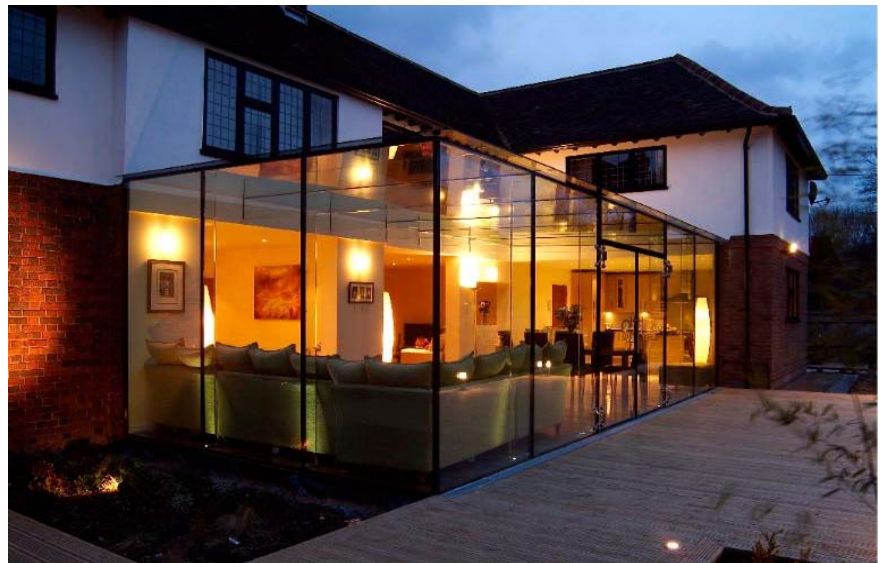
The new 9m long extension in Harpenden, opens up 1930s living spaces
