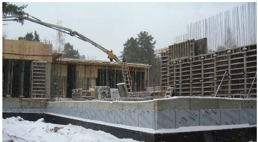
A special waterproofing membrane has been used for the basement foundations.
